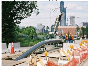
Improved PE Gas Pipe for Natural Gas Distribution - Bimodal PE2708 Gas Pipe Application
